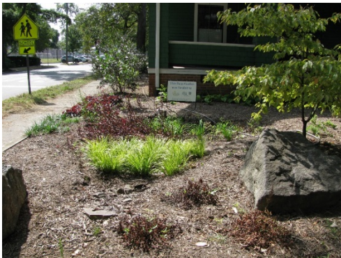
Image from City of Durham showing a bioretention cell retrofit.
