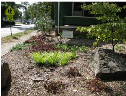
Image from City of Durham showing a bioretention cell retrofit.
