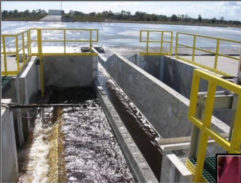
Harvested algae is conveyed to a concrete spillway.
