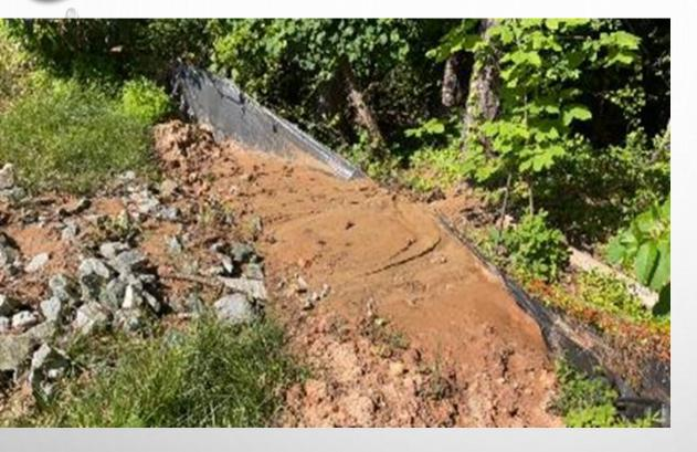
Silt fences help reduce sediment but must be installed properly and maintained – this is "offsite sediment" and is a violation.
