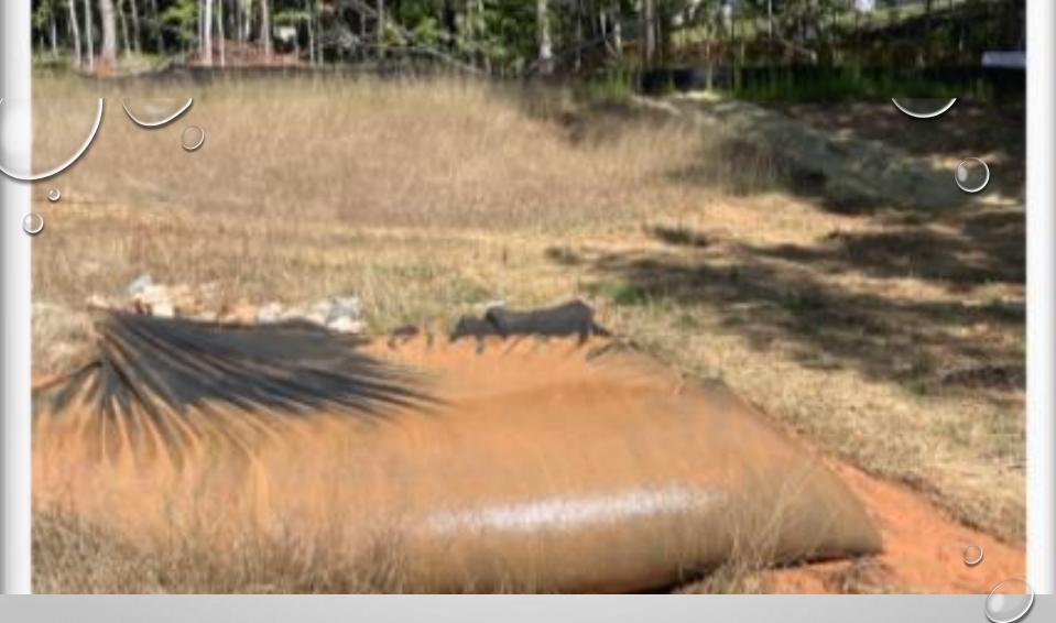
Sediment filter bags remove sediment, but effluent is still turbid due to particle size.
